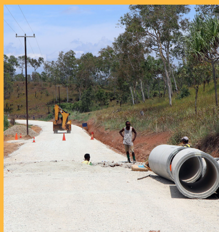
Locals engage with road contractor, Global Construction, to install culverts in the road.
